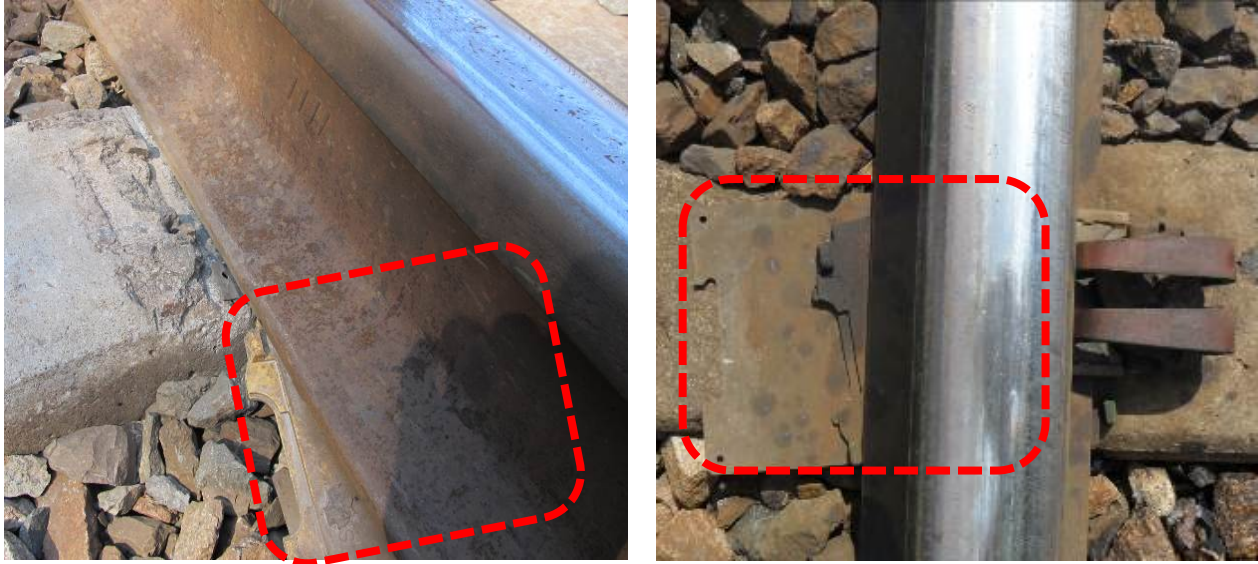
Figure 2.5 Examples of rail pad assemblies “walking out” of the rail seat
