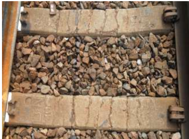
Figure 3.2 Cracked concrete crosstie due to center binding
