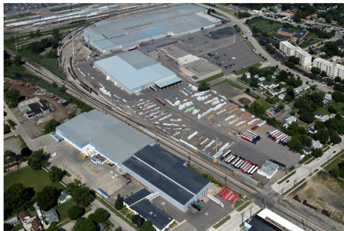
Figure 1 - Wayne Industries Steel Facility with rail access
