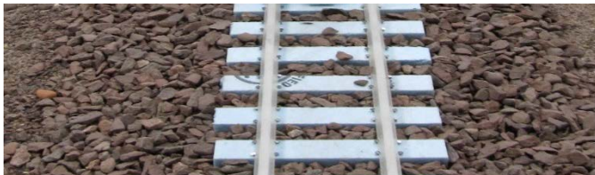
Figure 3. Track calculations and finished construction.
