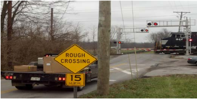
Figure 1. Brannon road crossing.
