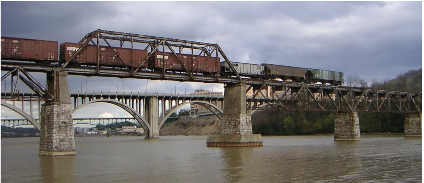
Research at UTK is expected to contribute on the seismic capacity assessment of thousands of existing stone masonry and unreinforced concrete railroad bridge piers.
