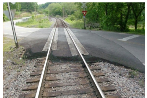
Typical Timber/Asphalt Crossing Surface
