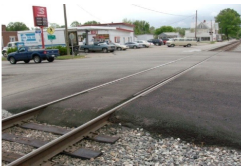
Typical Rubber Seal/Asphalt Crossing Surface
